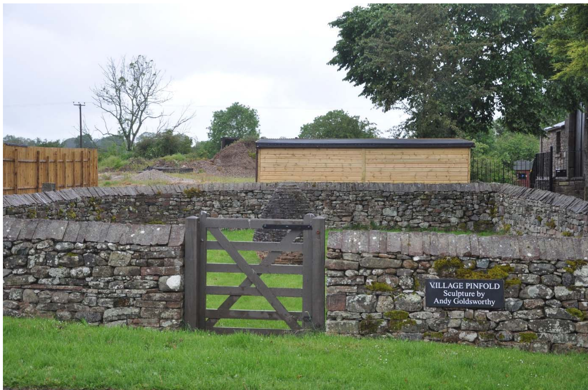
The structure complements the original pinfold in Bolton which contains a cairn by the celebrated sculptor Andy Goldsworthy.
